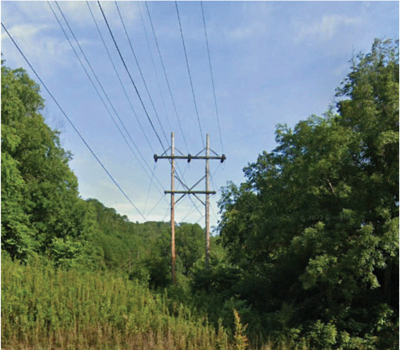
Existing Fieldale - West Bassett No. 2 69-kV Line H-Frame
