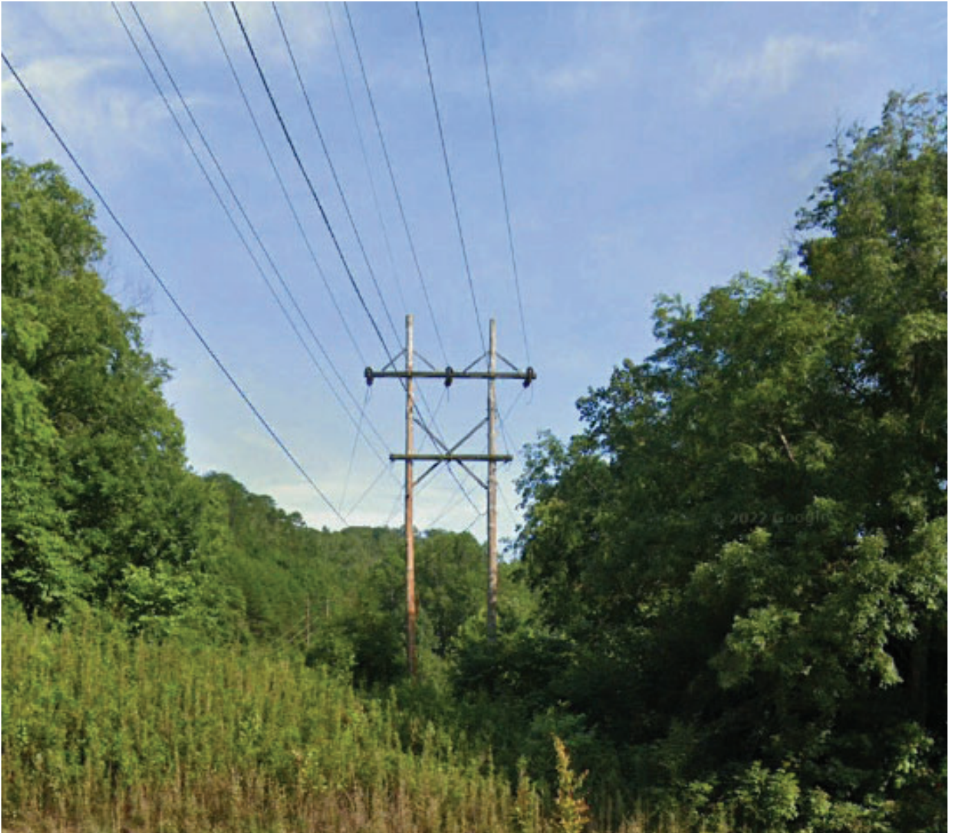
Existing Fieldale - West Bassett No. 1 69-kV Line H-Frame
