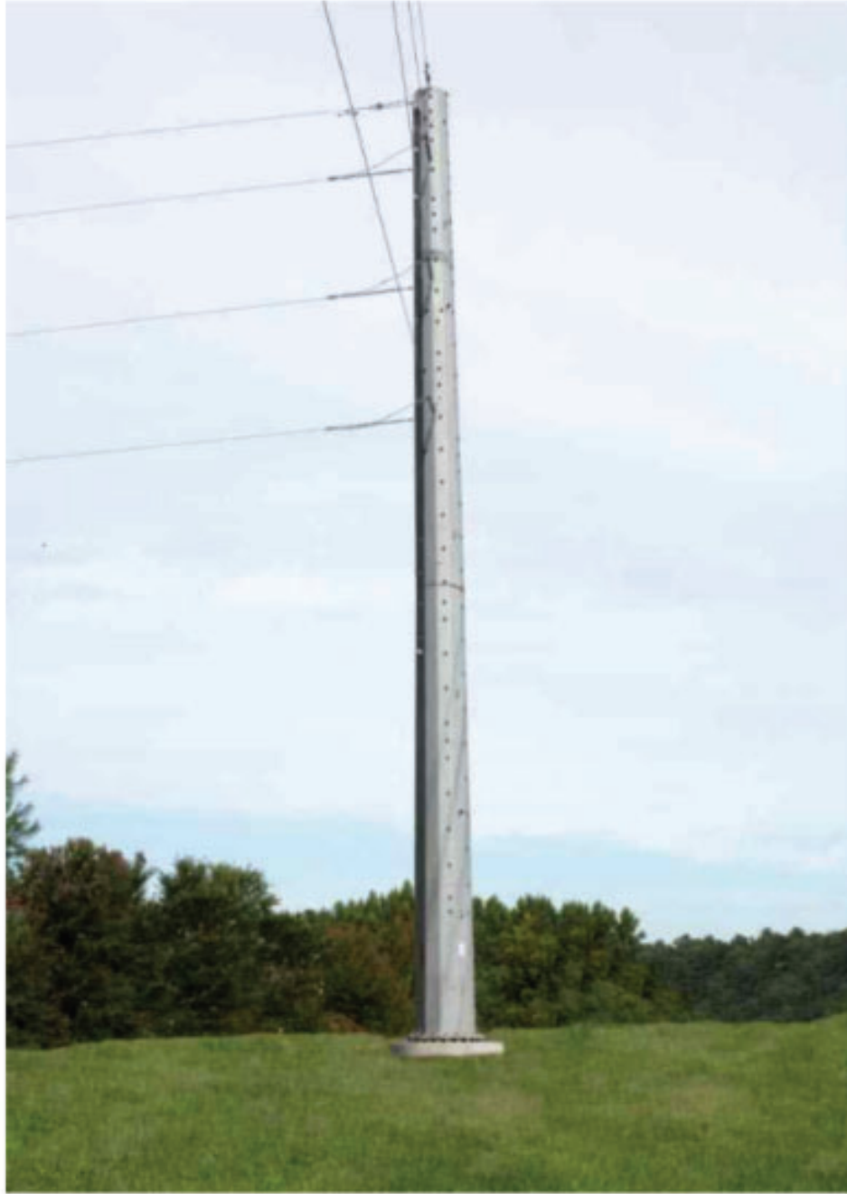
COMPARABLE EXISTING STRUCTURE PHOTOGRAPH
