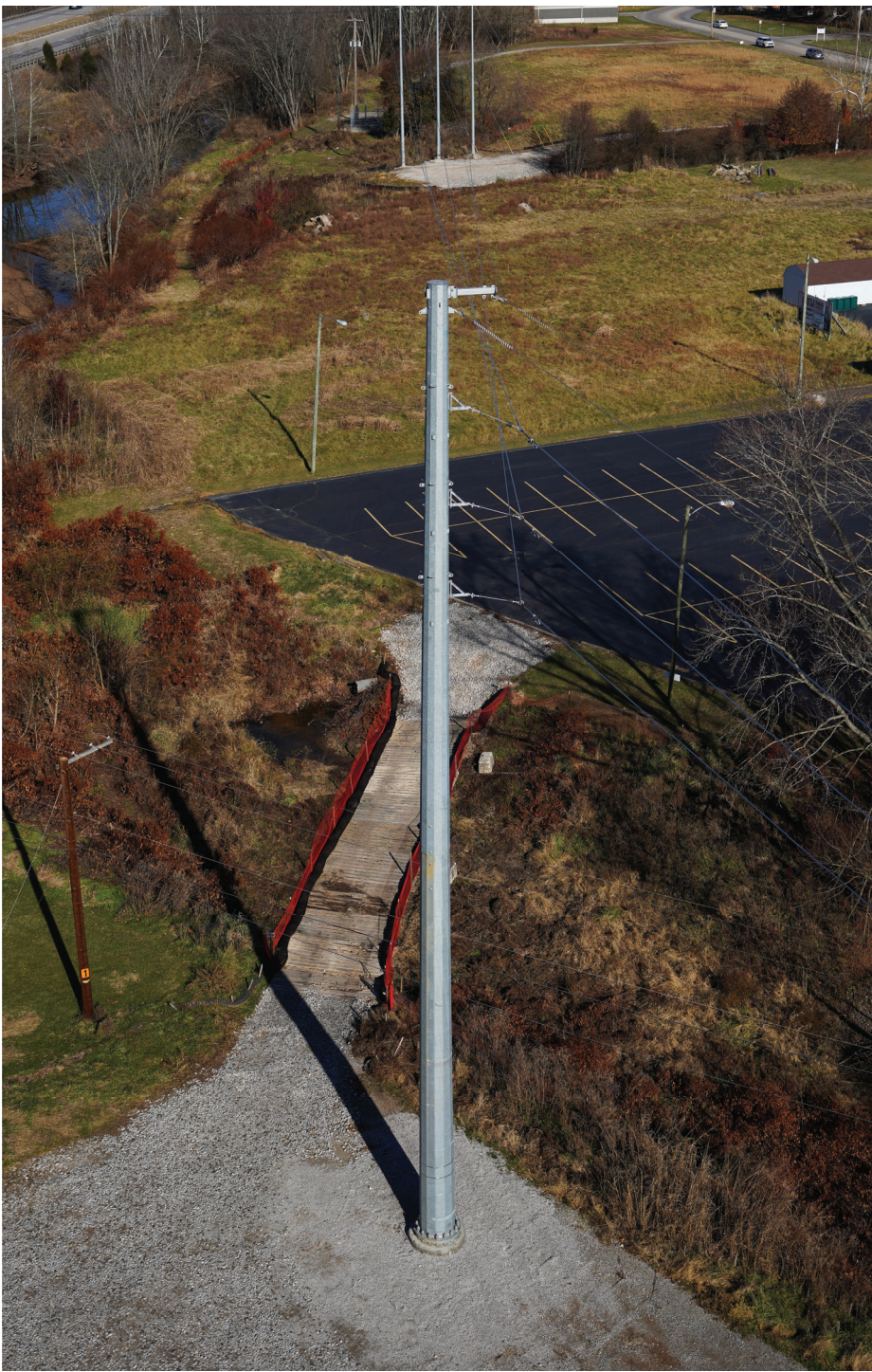
COMPARABLE EXISTING STRUCTURE PHOTOGRAPH
